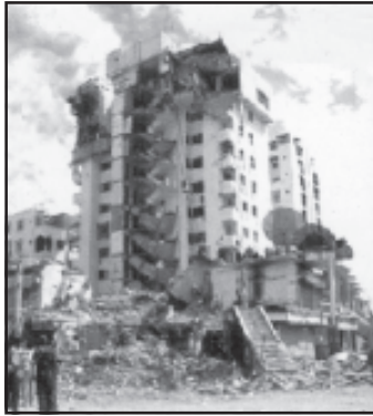
Fig. 3.3a: Destruction caused by an Earthquake in Gujarat
