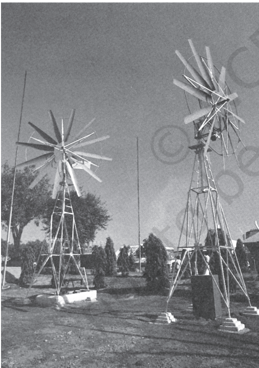
Fig. 8.7 Wind mill : another source of generating power
