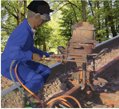
Figure 3.11 Thermit process for joining railway tracks
