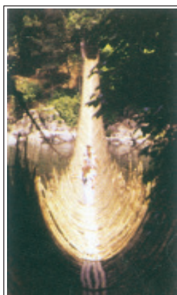
Figure 6.7 : Rope Bridge (Arunachal Pradesh)
