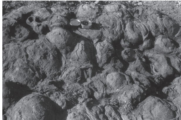
Fig.6.4 : Exfoliation (Flaking) and granular disintegration
