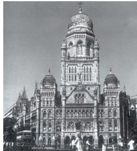
Fig. 12.29 The Municipal Corporation Building, Bombay, designed by F. W. Stevens in 1888
